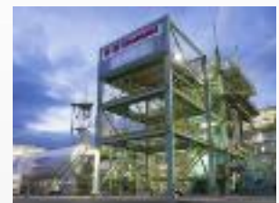
Hydrogen Liquefaction Facility
